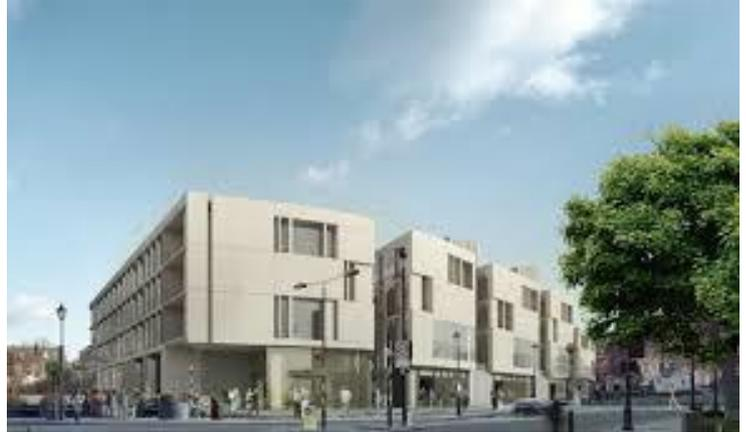
This was neither practical nor cost effective in the primary Jura limestone, or in matching pre-cast concrete due to casting and weight issues. It was therefore decided early within the design process this could only be constructed in glass reinforced concrete.
