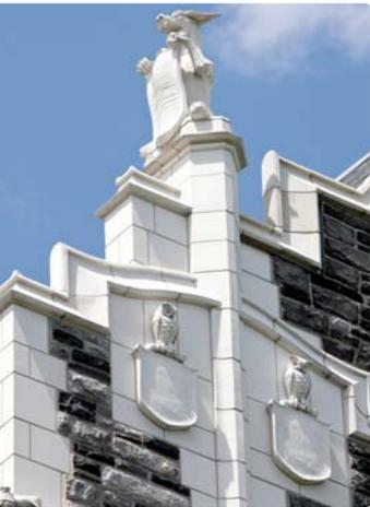
GRC replaced the original cladding during restoration work on Sheppard Hall at New York's Central College.
