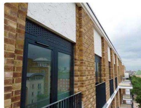
**Large-scale GRC cladding panels at entrance, balcony and roof level, which feature a repeating Canadian maple leaf design.**
